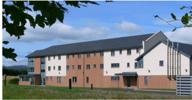
New £3.5m boarding house at Glenalmond College
