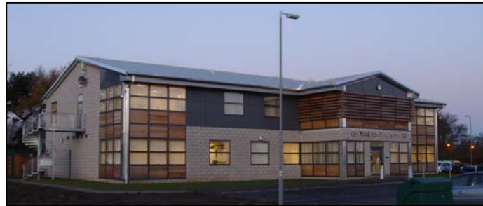
New build £1.8m police facility for Central Scotland Police
