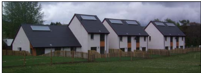
10 new houses at Sillerburn, Kirkmichael for Perthshire HA
